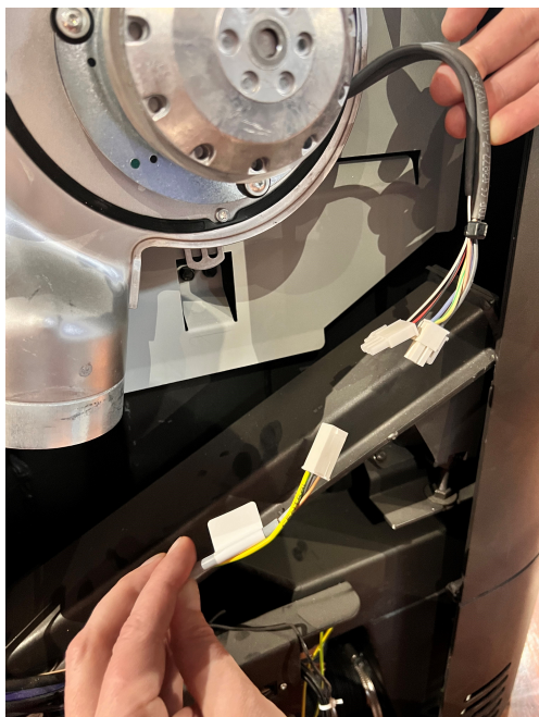
Fig. 47: Connecting the cables
